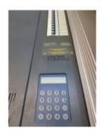
Step 9: Check that the MCB (Miniature Circuit Breakers) are turned ON, there is power to the Dimmers, do this ONLY if you are authorised to do it, AS THE DIMMERS COULD BE FAULTY AND ARE SHUT DOWN OR PEOPLE ARE WORKING ON THE DIMMERS
